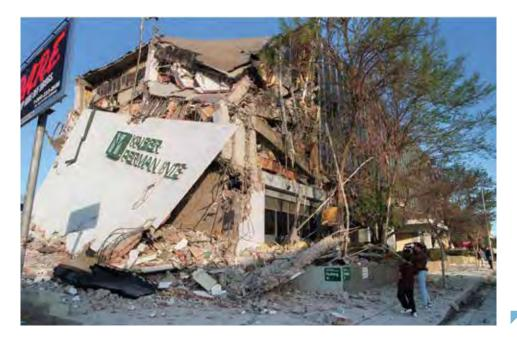
Older non-ductile concrete buildings were constructed using more brittle material, making them hazardous in an earthquake.
